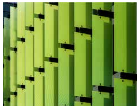
Creative Campus Parking Structure
